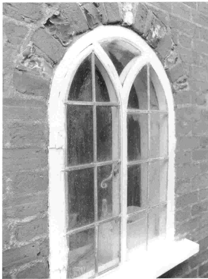
FIG. 127 – The ground-floor window at Stoke Ash.
