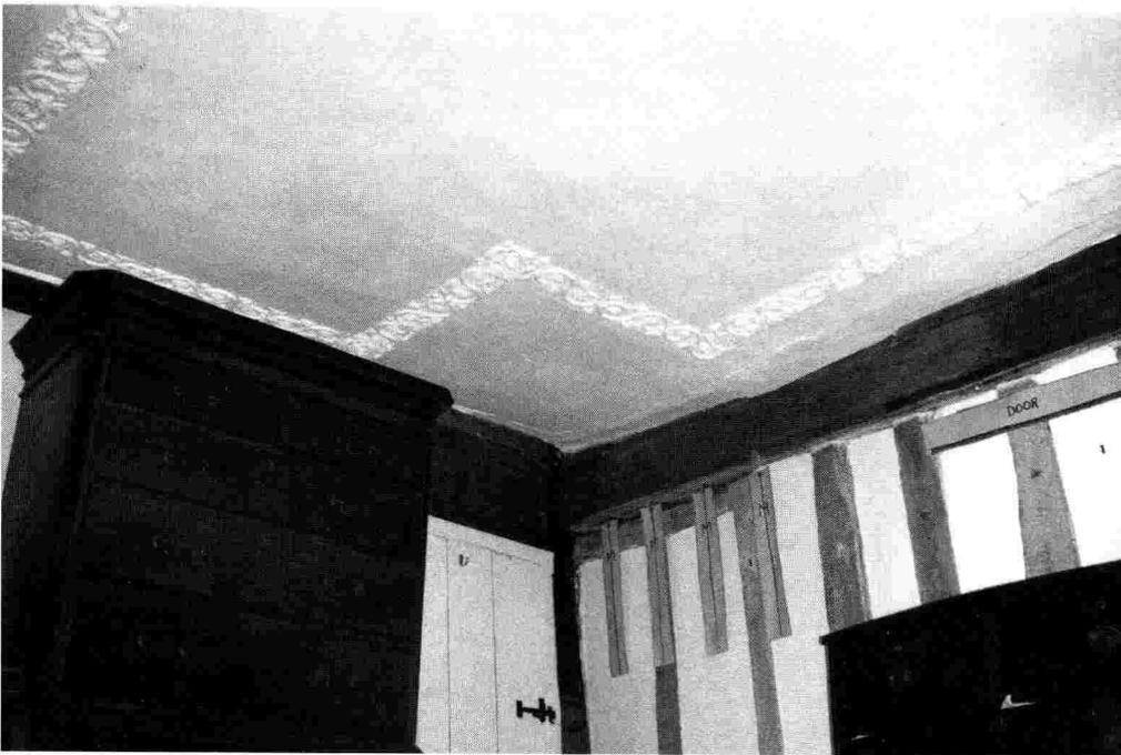
Boundary Farm: N.W. corner of the parlour chamber, showing the positions of the 1st phase window (mullions indicated by vertical card strips), 2nd phase door (indicated by horizontal card strip) and ceiling evidence for 3rd phase internal porch.
