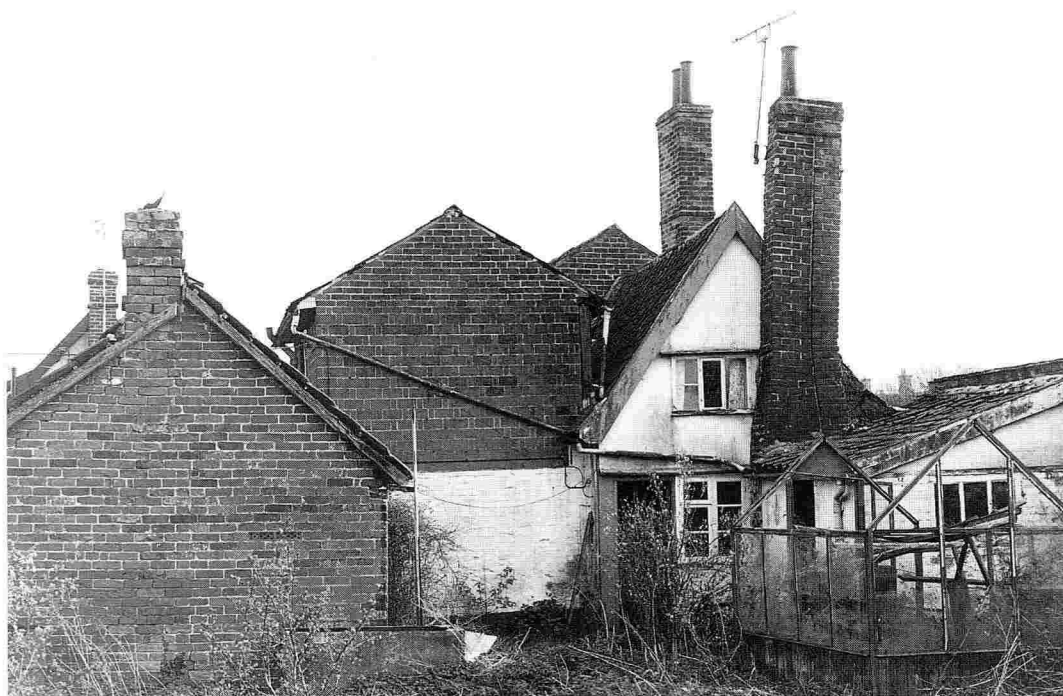
FIG. 145 – North gable of cottage and cell block with rat-trap bonded brickwork on upper floor. Wash-house to right and garden building with chimney on left ( photo: author ).
