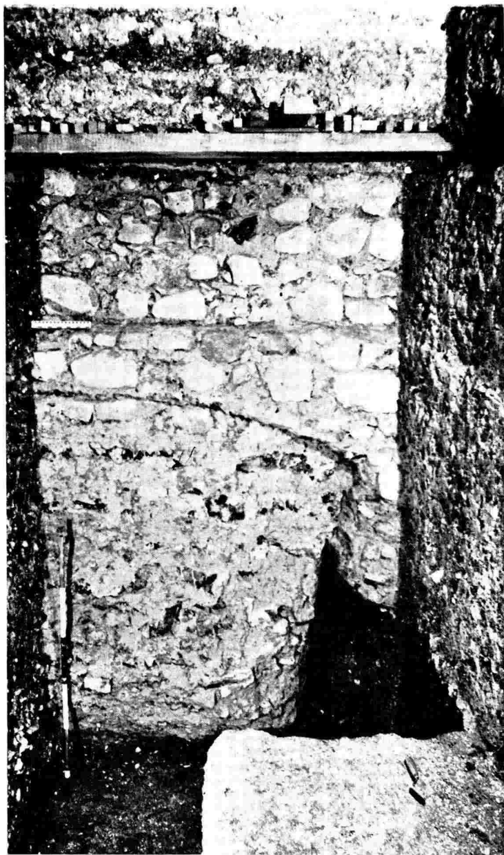
Foundation of part of the curtain wall, showing the clear difference between the face-built and trench-built parts. The shored-up wall at the top belongs to the later Poor House.
