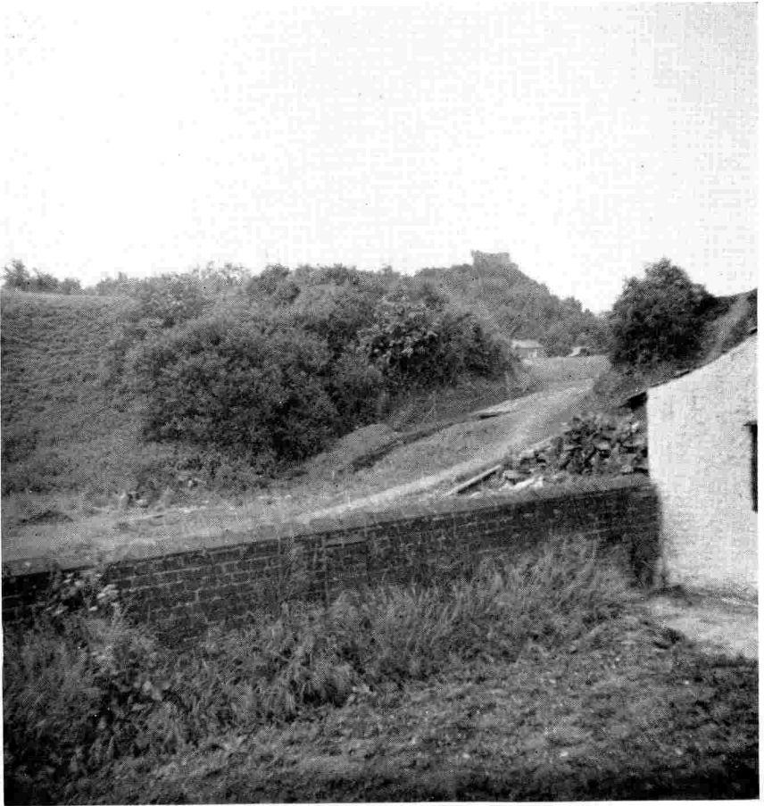
Entrance to outer bailey, Clare Castle, looking towards the motte
