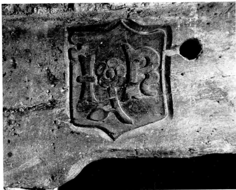
Shield at left end of fireplace beam.
