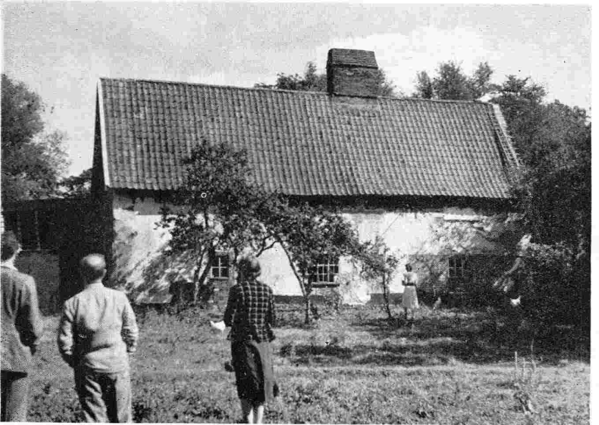
The roof partly repaired.
