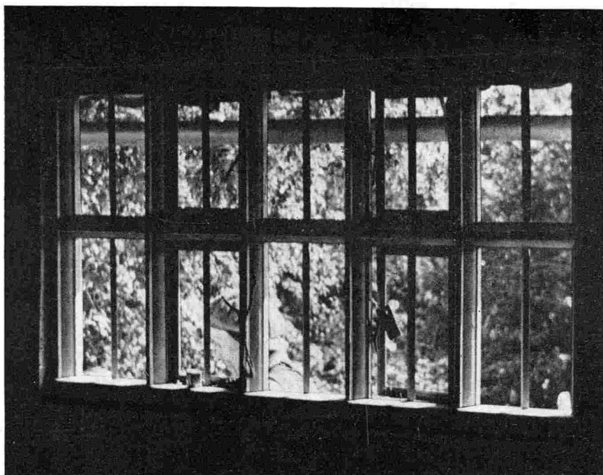
The new windows.
