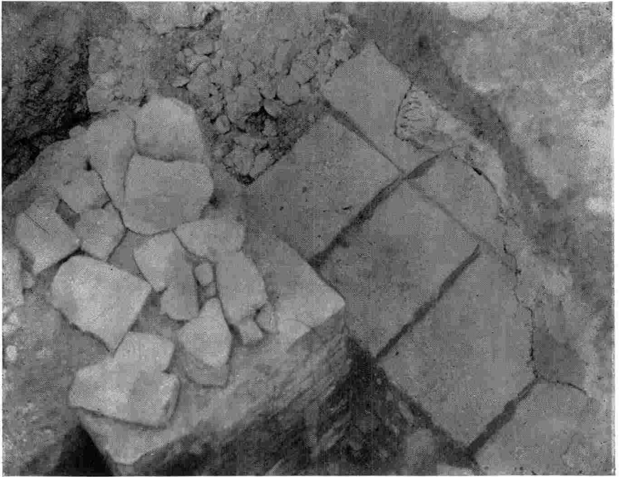
Fig. 2 Foundation of third brick buttress shewing stone-paved area, from the south east.
