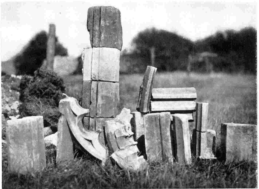
Fig 3. Some of the dressed stone work from the area to the north of the third buttress. Sections of drip moulding, mullion transoms, and window bead moulding are included.
