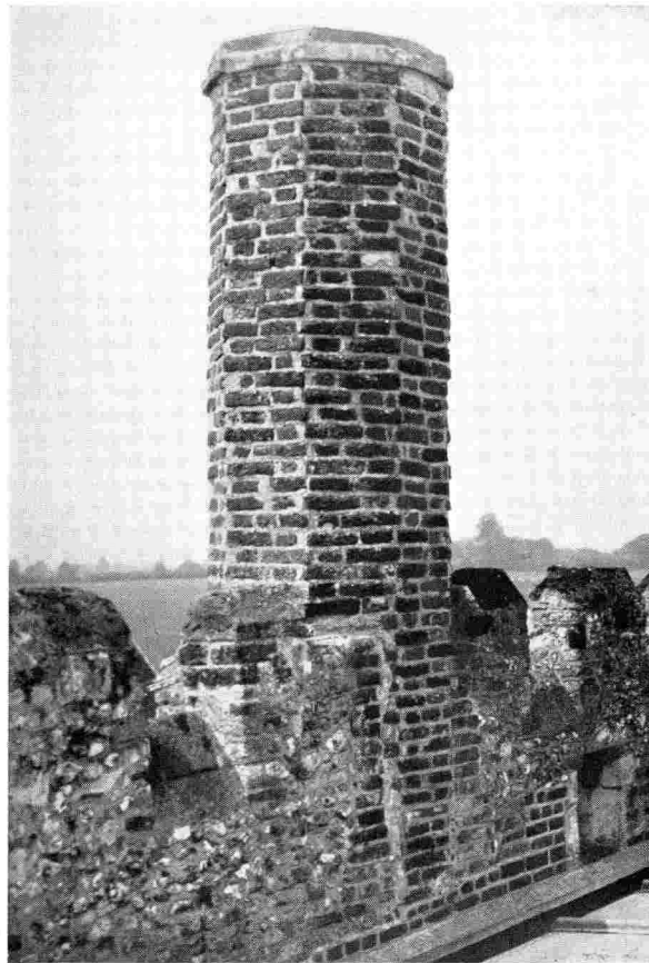
LITTLE WENHAM HALL, SUFFOLK. Octagonal brick chimney. Probably built about 1565-1569, when alterations and additions were made to the earlier building.
