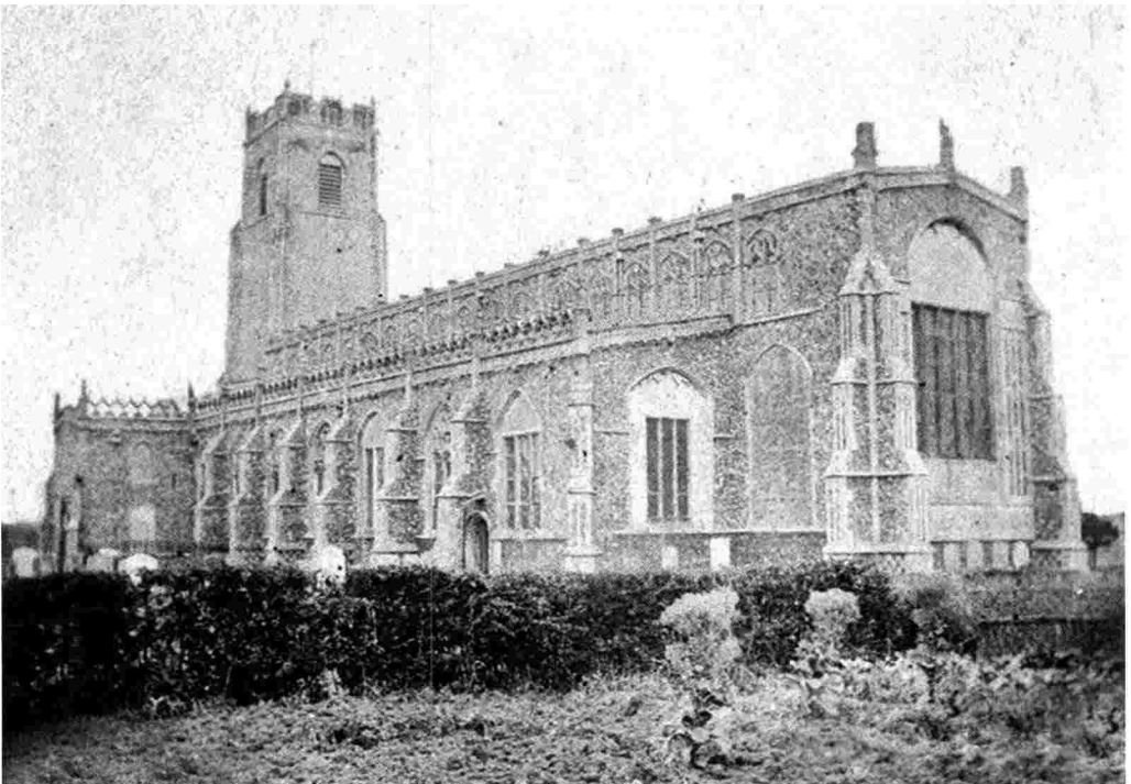
FIG. 142 – Blythburgh Church at about the time of Geldart’s visit ( Society for the Protection of Ancient Buildings ).
