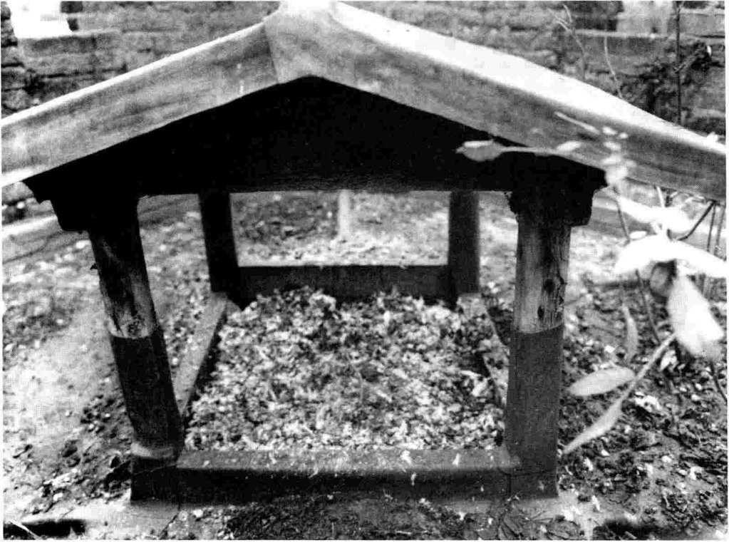
FIG. 6 – The louver on the roof of the turret, from the east ( photo: author ).
