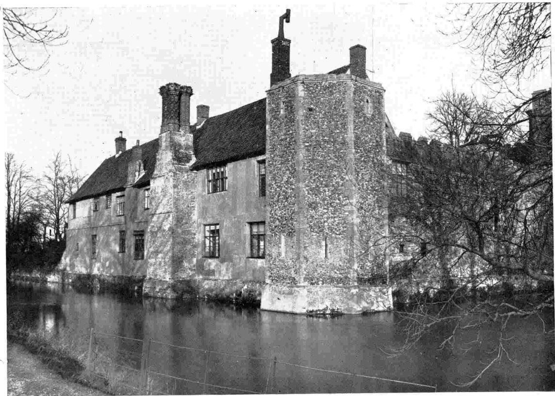
WINGFIELD CASTLE. SHOWING TUDOR HOUSE ON WEST SIDE.
