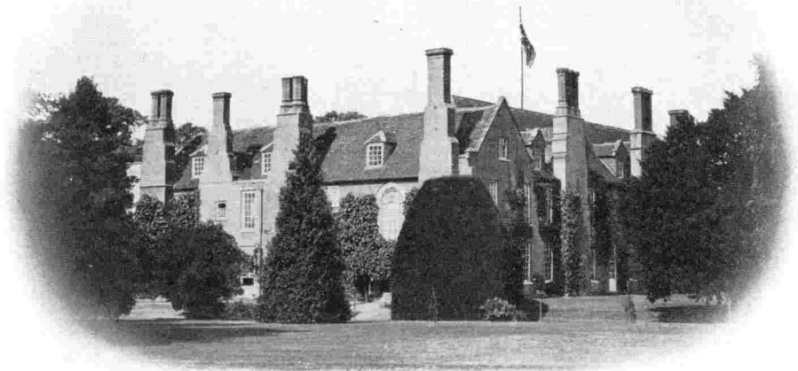
HINTLESHAM HALL: VIEW OF SOUTH EAST.
